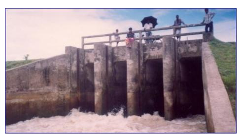
A Sluice Gate in Bera Upazila, Pabna. Timely Operation of Sluice Gates is necessary for Fish Migration into Floodplain Source: BCAS
