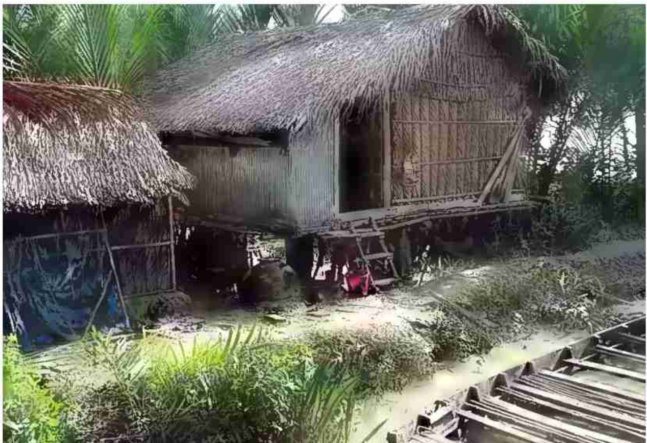
Coastal Communities are adapting to high tide & sea level rise with raised House
