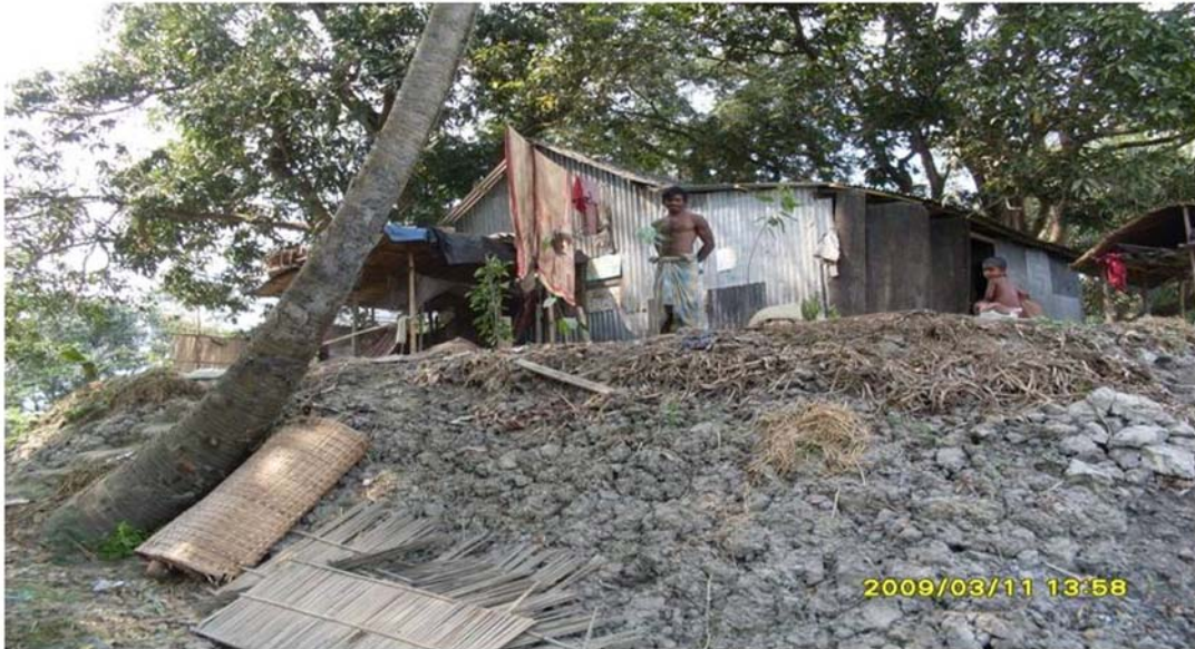
Homestead plinth raised in floor and water logging affected site, Muksudpur, Gopalganj district
