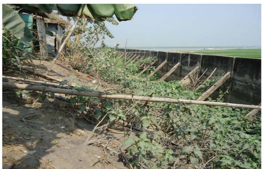
Village erosion protection wall in Nikly, Kishorganj district
