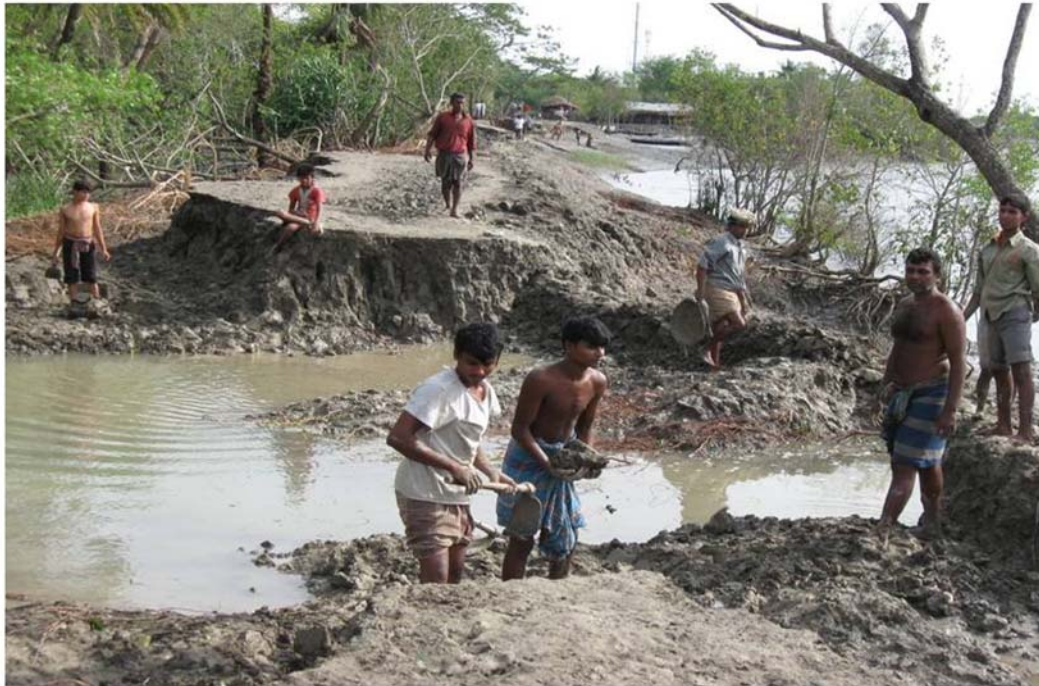
Community based initiative in re-building coastal embankment
